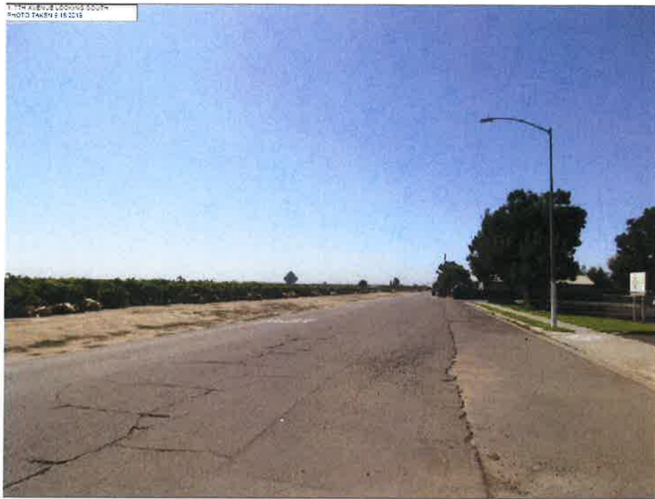
7 th Avenue looking South
