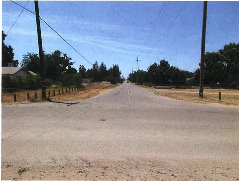
Ashlan Avenue looking West
