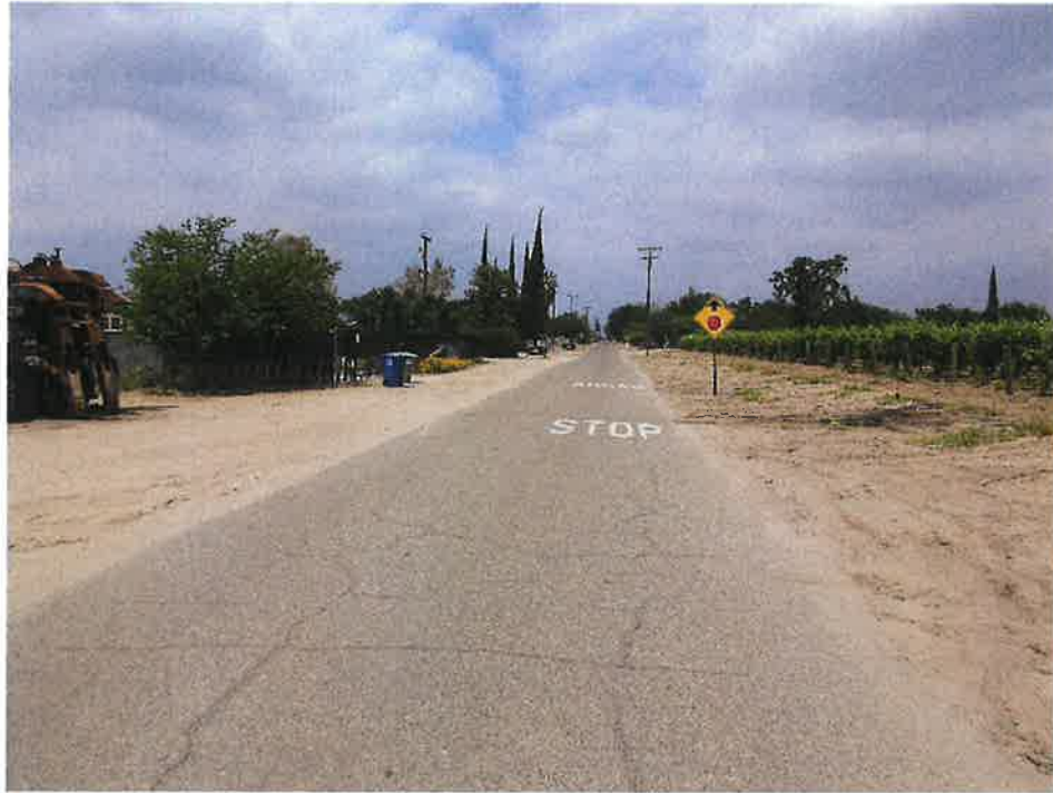
Floyd Avenue looking North (South of Church)
