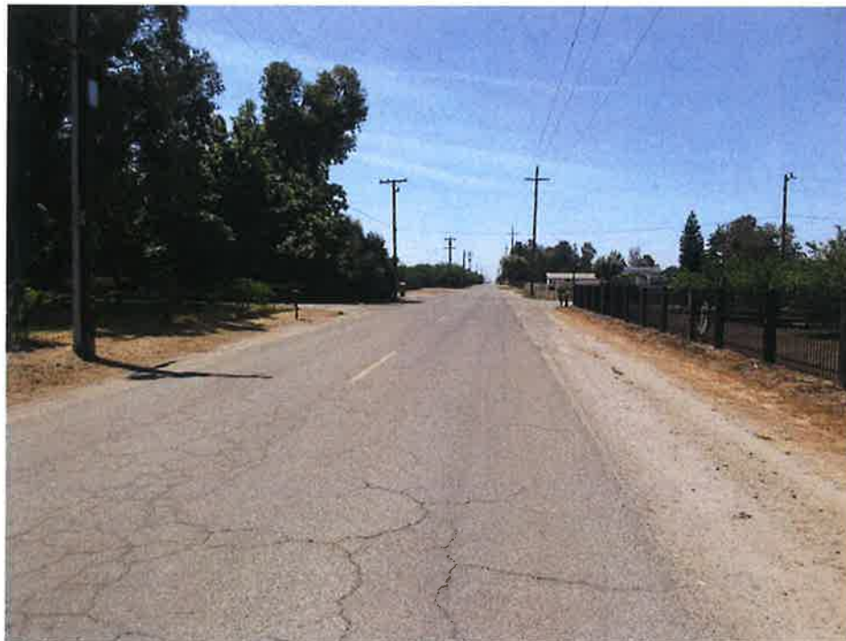
Ashlan Avenue looking West
