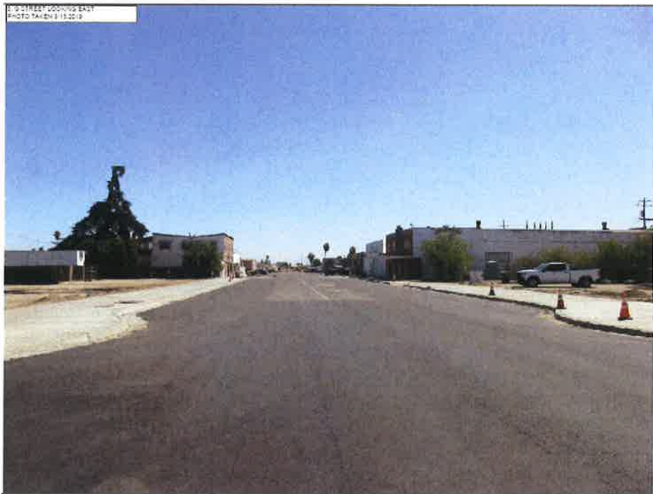
G Street looking East
