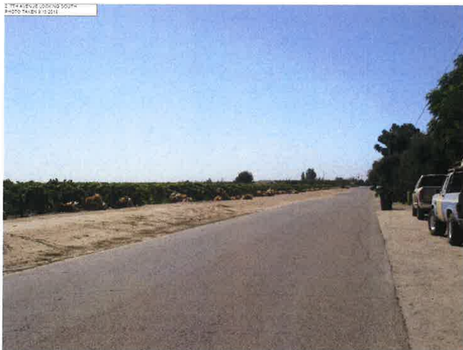
7 th Avenue looking South
