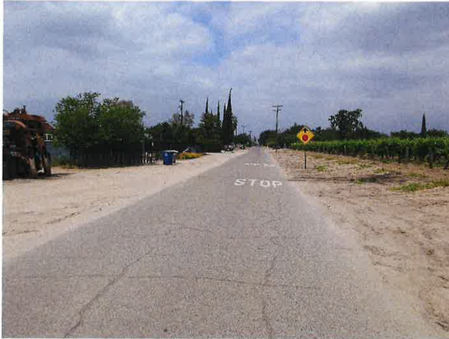
Floyd Avenue looking North (South of Church)
