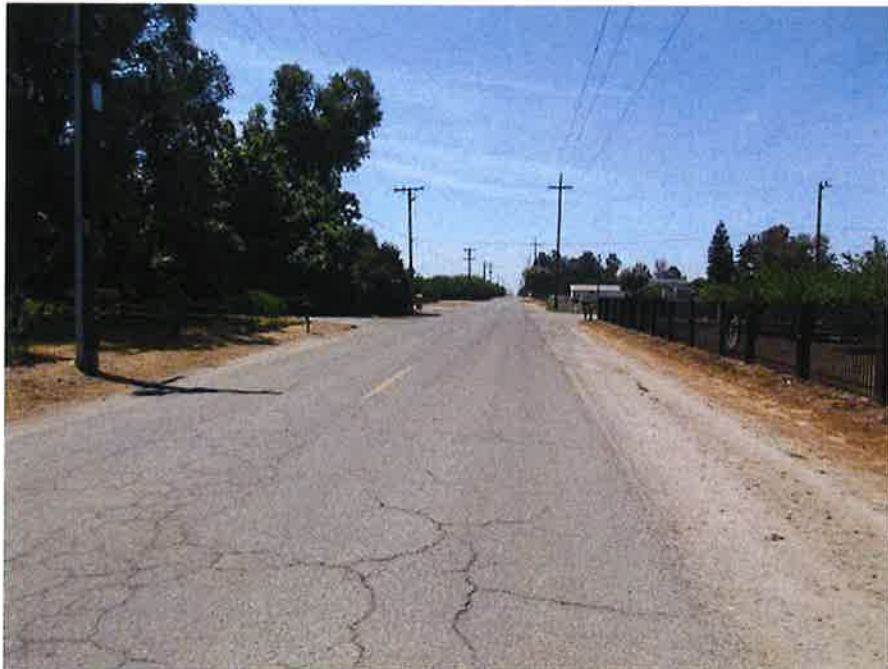
Ashlan Avenue looking West
