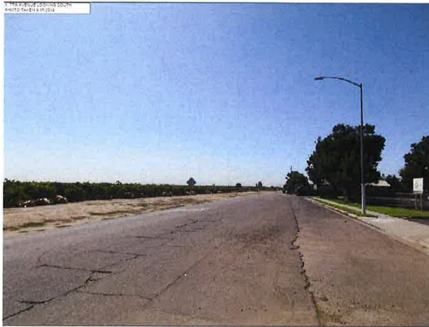
7 th Avenue looking South
